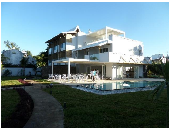
View of restaurant and SW-pool
